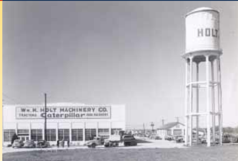
Wm. K. Holt Machinery Co. headquarters in San Antonio, Texas, leased from H.B. Zachry Company until 1957.
